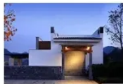
Household Energy Storage
